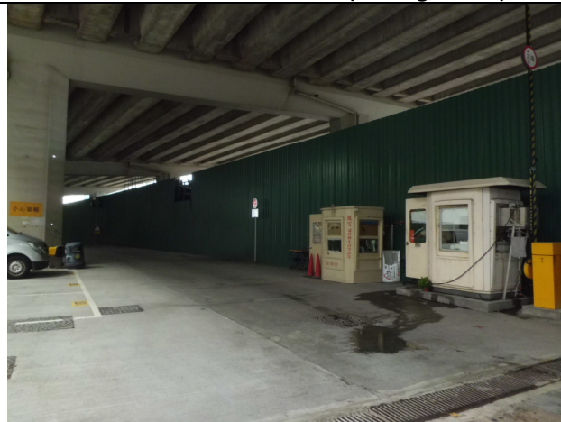
Photo 3 - FEHD (Between Victoria Centre and the project site)
