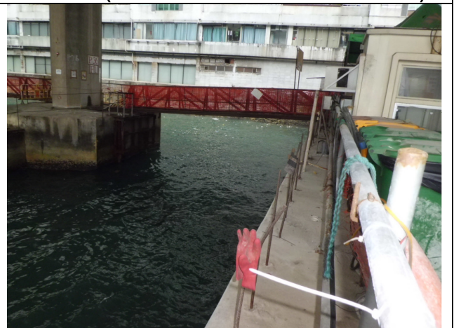
Photo 6 - Marine portion facing City Garden
